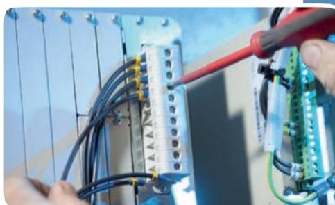
Arc protection systems require three phase currents for selective high-speed arc protection. Using the zero-sequence voltage and current in tripping criteria, the arc fault trip can be activated before the fault is completely exposed.
