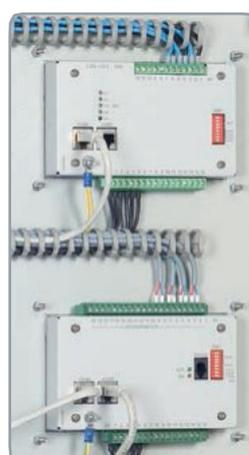
Door mounted I/O units show arc protection system information without opening the secondary compartment door
