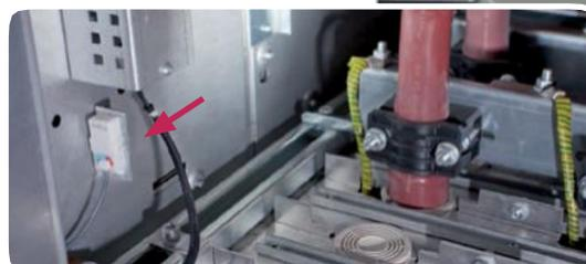
The majority of arc faults occur in the cable compartment hence it is a natural location for the point sensor.
